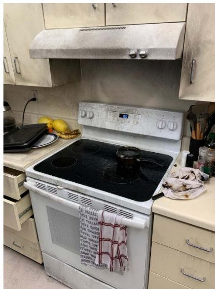
Stove Top Cooking Fire Damage
