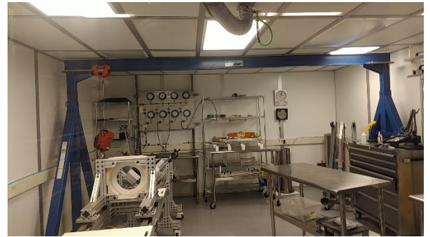
Figure 4: Portable gantry crane with manual chain hoist
