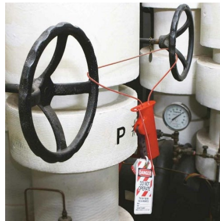
Valve lockout with cable Brady.com
