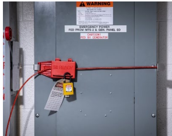
Panel lockout with cable Brady.com
