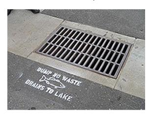
Stormwater drains connect to underground sewer pipes that carry water and anything picked up along way directly to the nearest body of water:
