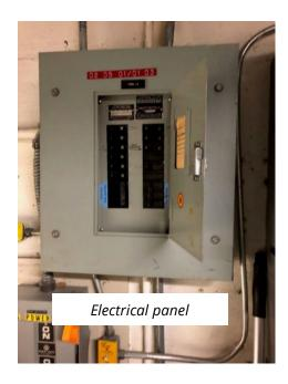
Before resetting a breaker, you *must determine the* cause of the trip. It is safe to reset a breaker only if it has been determined that the circuit was overloaded. Repeatedly resetting a breaker could result in an arc flash or a fire.
