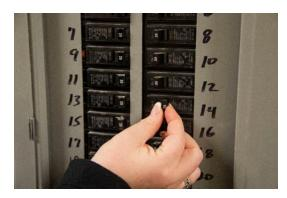
Stand to the side of the panel and use one hand to flip the breaker from the "off" position to "on."
