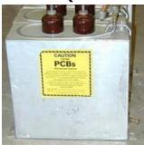
Other types of older oil-filled electrical equipment must be removed and/or replaced whenever feasible and disposed of properly through EH&S.
